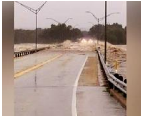
Collapse of old FM 2900 Bridge
