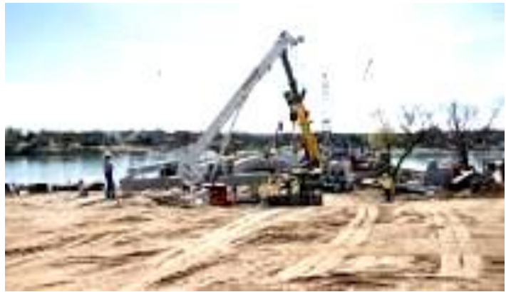
First 80 ft span beam being laid at site of new Bridge
