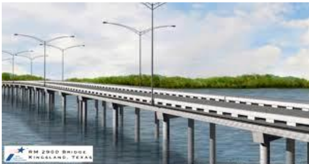
Picture of future $17.3 Million RM 2900 Bridge (to be completed in April, 2019)
